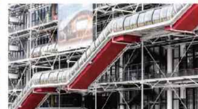
Steel Structure Industry
