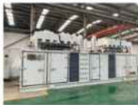
内蒙古某砖井站项目 Inner mongolia brick well station project
