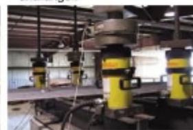
▲ Synchronous lifting of steel structure in gymnasium construction.
